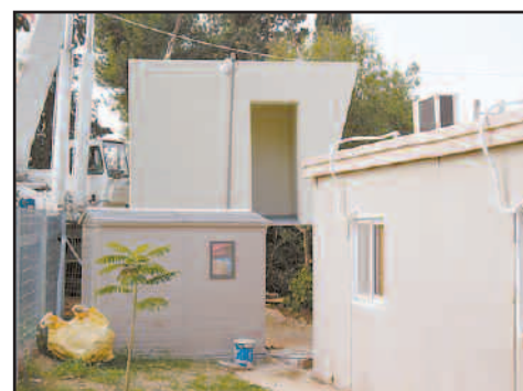
Shelter being lowered behind kindergarten.
